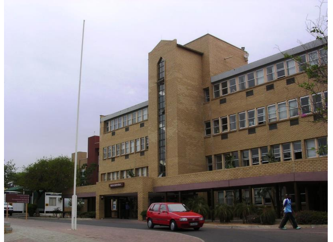
Princess Marina Hospital—opened in 1967— 4 operating rooms—principal referral hospital for country
